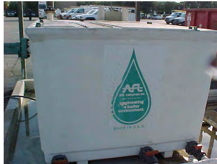
Above-ground oil/water separator
