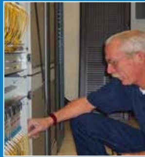
TRANSPORT EQUIPMENT INSTALLATION
